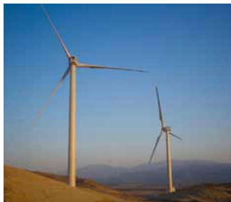
▲ BP owns and operates the Edom Hills wind farm in Southern California.
