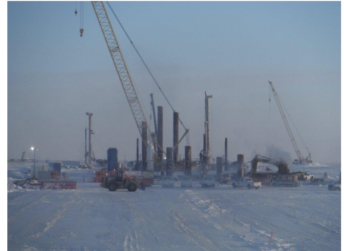
CD5 Construction Activities
