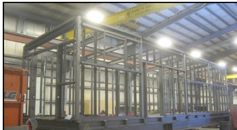
Nana Construction: Airstrip Regulator Shelter Big Lake, AK
