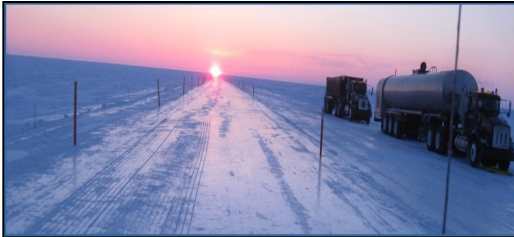
Ice road construction
